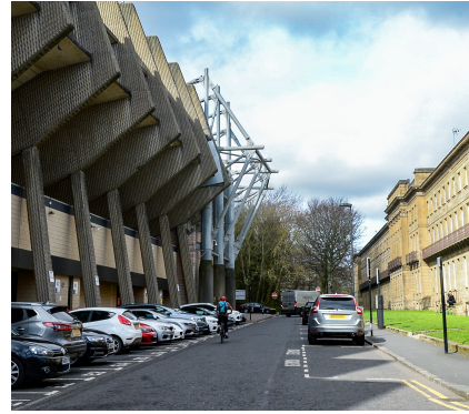
Figure 5. Leazes Terrace adjacent to the East Stand
