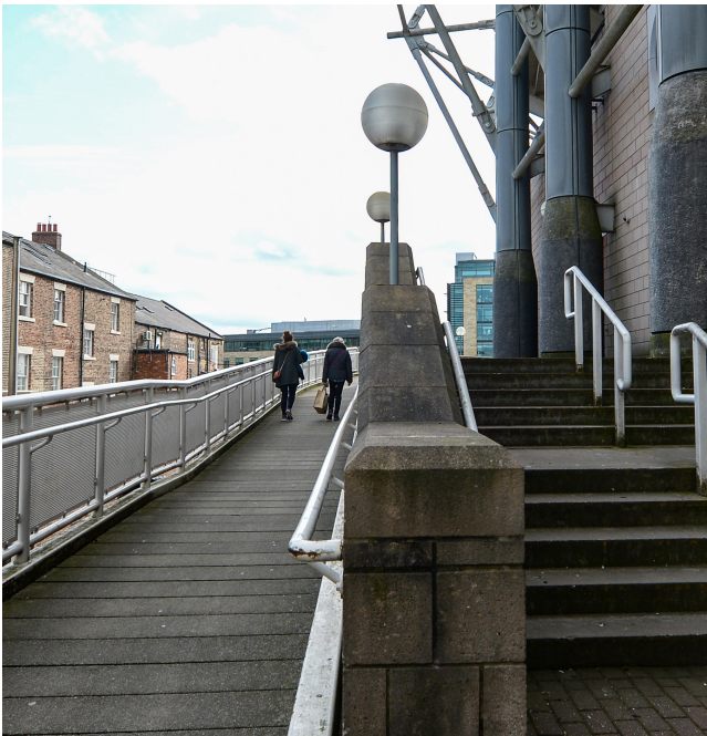
Figure 11. Access ramp located in the South East corner
